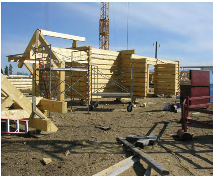
Dovetail construction
