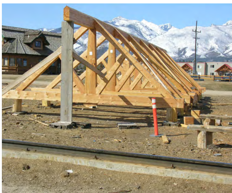
Timber roof structure
