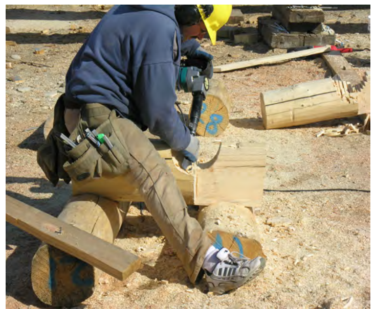
Notching a hand-scribed saddle notch
