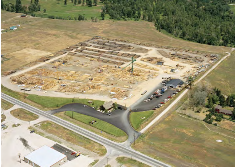
Aerial view of Pioneer Log Homes crafting yard in Victor, MT
