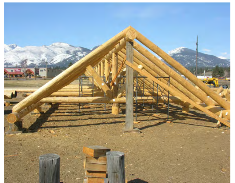
Completed log roof section
